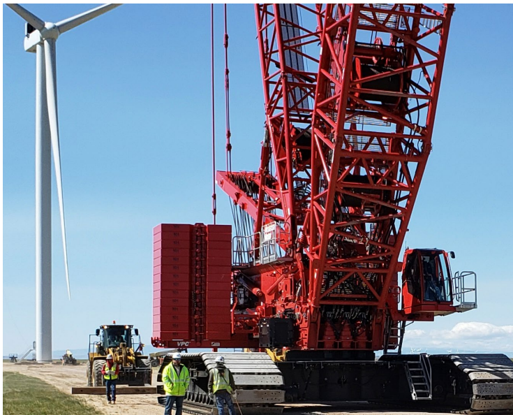
Figure 1. Crane walking to a new wind turbine site 2 .
